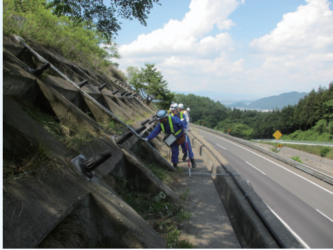
切土のり面の点検
