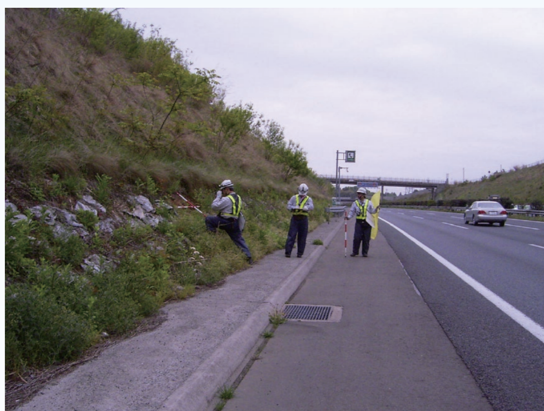
切土のり面の点検
