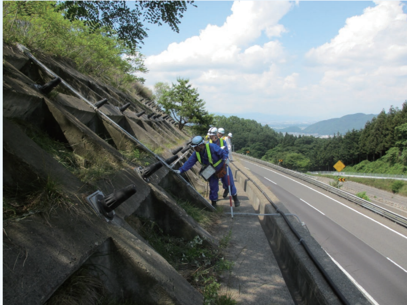
切土のり面の点検
