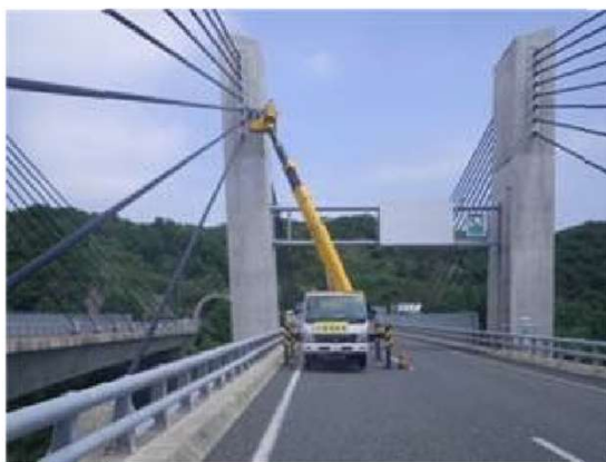
橋梁の近接目視点検
