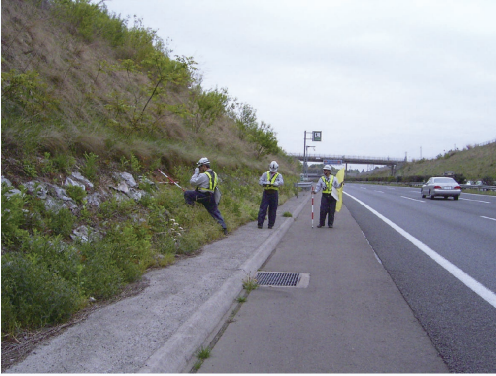
切土のり面の点検
