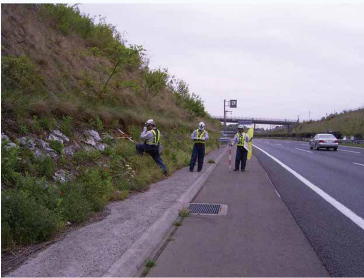
切土のり面の点検
