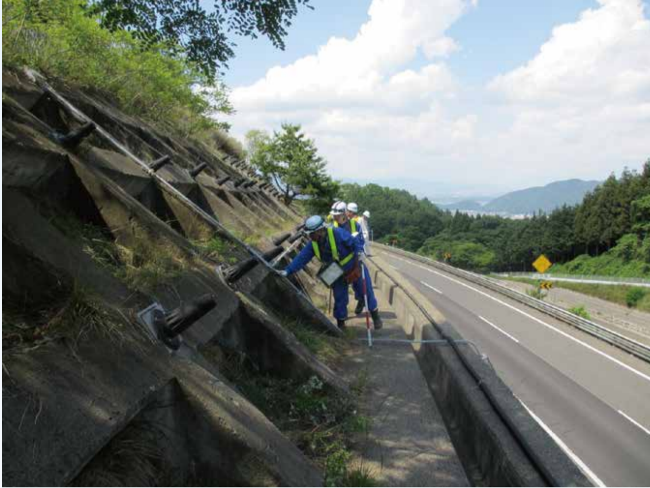
切土のり面の点検
